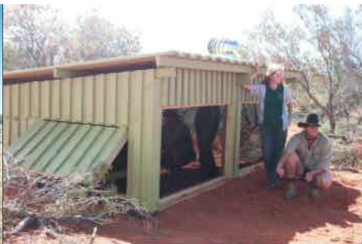
The above and below-ground viewing hide built within the First Expansion area. Tours to the Reserve will begin in 2002.
